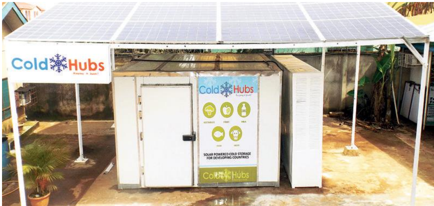
ColdHubs has installed solar-powered walk-in refrigeration units like these near farms and markets COLDHUBS
