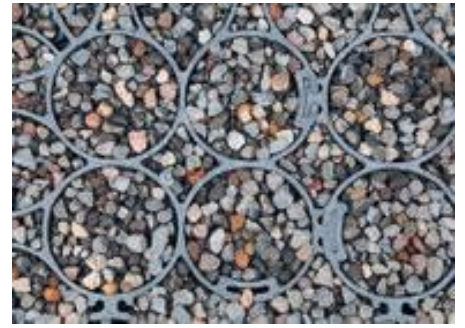
Gravalock grids have been used in 40,000 sq m of industrial parks and housing complexes
